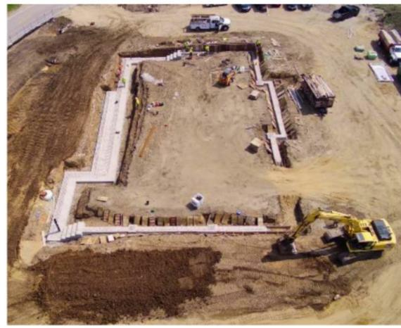
Work, to date, includes excavation and pouring of the foundation. The excavation activity prepared the earth for the building, the eventual parking area and the landscaping for water retention. The foundation work included installing forms and
